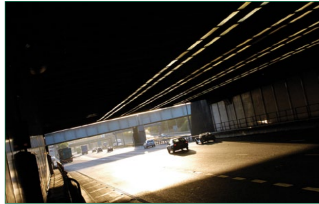
Holmesdale Tunnel United Kingdom
